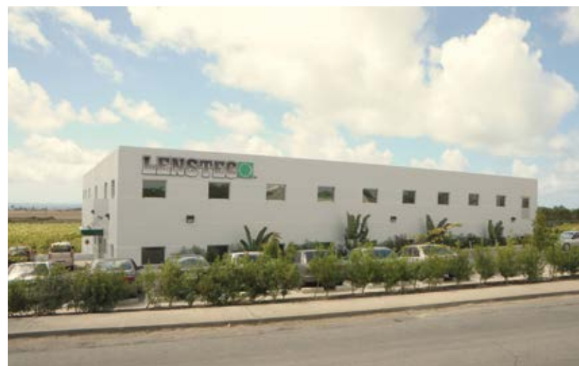
Lenstec Inc. Barbados manufacturing facility
