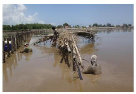
Figure 6.12 Placing the filling material between the walaba poles (Source: Naipal, 2015)
