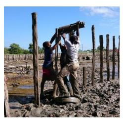
Figure 6.11 Slamming the walaba poles into the soil (Source: Naipal, 2015)
